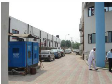
Multiline 200 kVA rental diesel generator installed on the premises of a multinational company near Lahore
